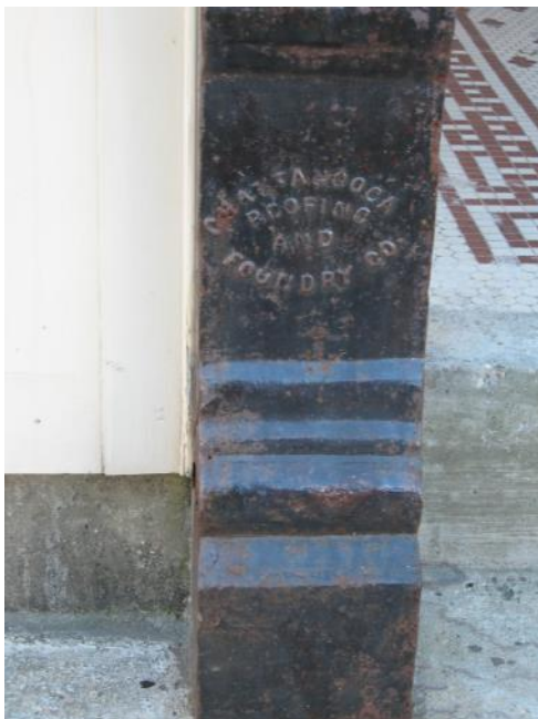
Details such as cast iron and entrance floor are also significant architectural features and should not be removed or concealed (119 Concord Street).
