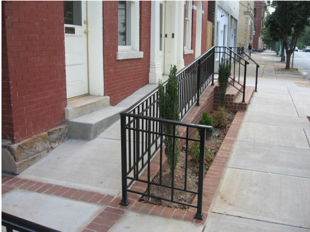
This ramp is appropriately designed for the front of this commercial building.
