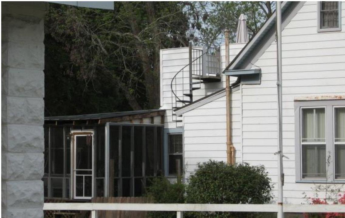
This exterior staircase is appropriately sited at the rear of the house with limited visibility from the street. Its spiral form helps to minimize visibility and its metal construction is appropriate.
