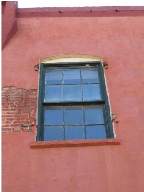
This original six-over-six sash window remains on the Wise Building at 315 Pere Megret. The historic photo shows not only the window but also its original shutters. Replacing the shutters is encouraged to help protect the window from the elements.
