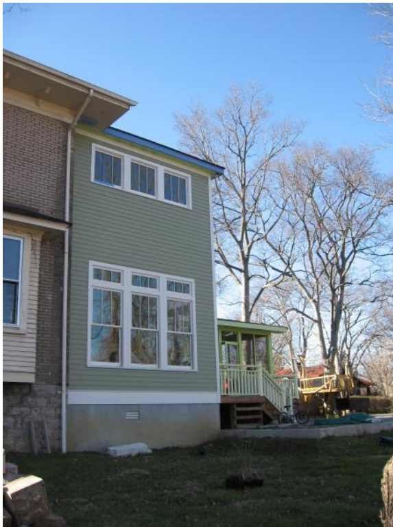
At left is an example of an appropriately scaled and designed addition at the rear of a historic dwelling. At right are appropriately placed and sized dormer additions on a rear elevation.
