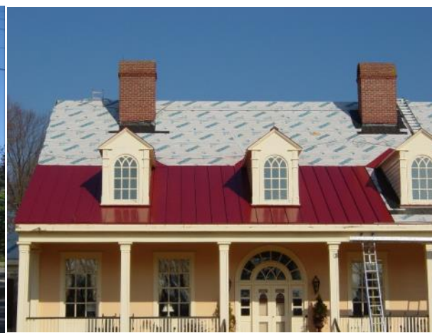
Original side gable roof forms should not be altered as at the Bungalow dwelling at 213 S. Main Street. New metal roofs should be of appropriate crimping and spacing as shown at the right.
