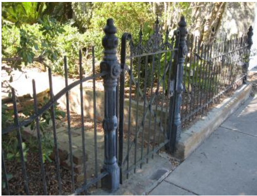
Historic fences in the district should be preserved and maintained such as the cast iron fence at 132 S. Main Street.
