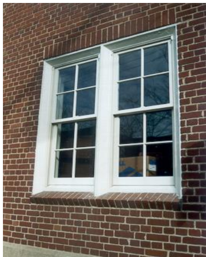
This original six-over-six sash window remains on the Wise Building at 315 Pere Megret. The historic photo shows not only the window but also its original shutters. Replacing the shutters is encouraged to help protect the window from the elements.
