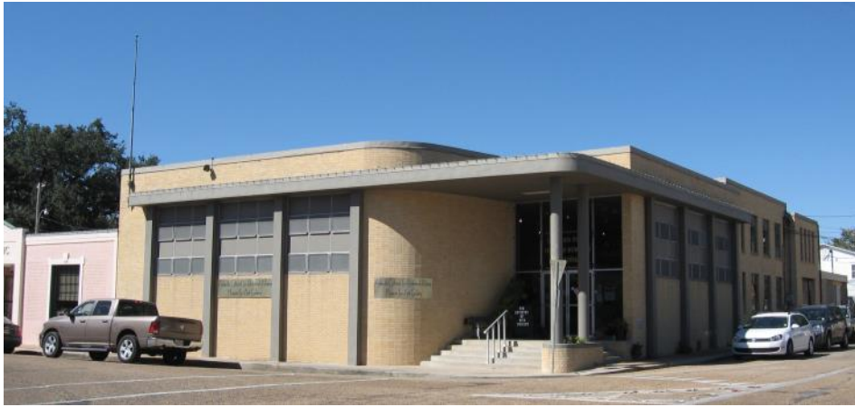
Historically unpainted brick should remain unpainted such as the Art Moderne style building at 200 N. Magdalen Square.
